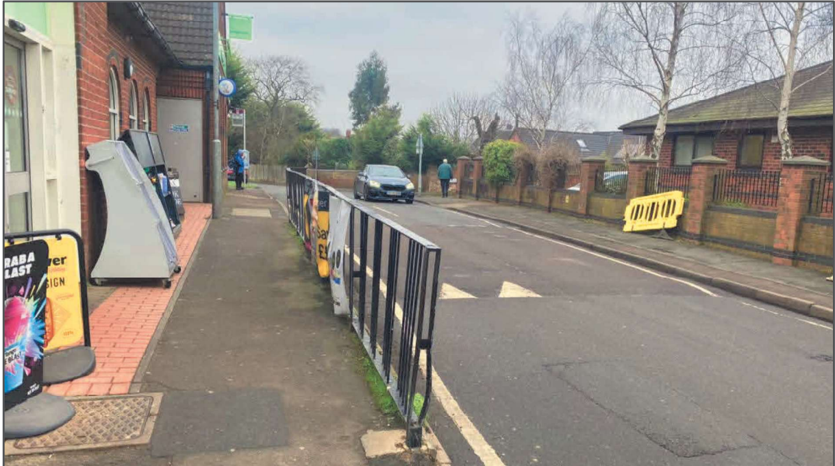
Figure 17 – High Street Raised Table
