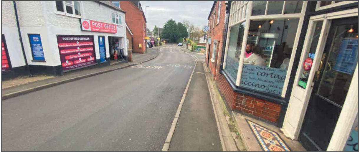
Figure 12 – High Street Footway
